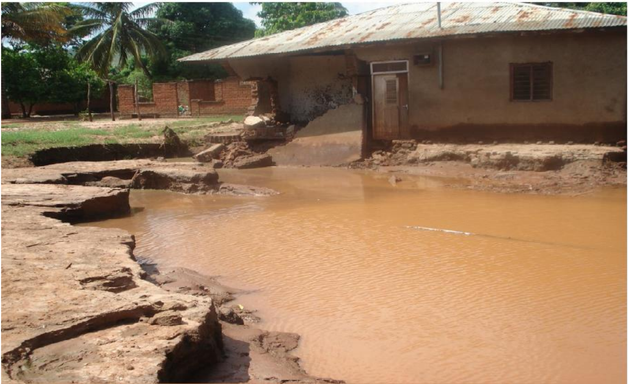
Plate 1: Flood impacts in Kilosa Township, February 2010.
